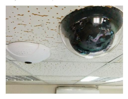
With the flexible and comprehensive Trigger Policy and Motion Detection provided by Genius Vision NVR, a panorama camera can be used to guide a speed dome, by calling preset points upon motion.
